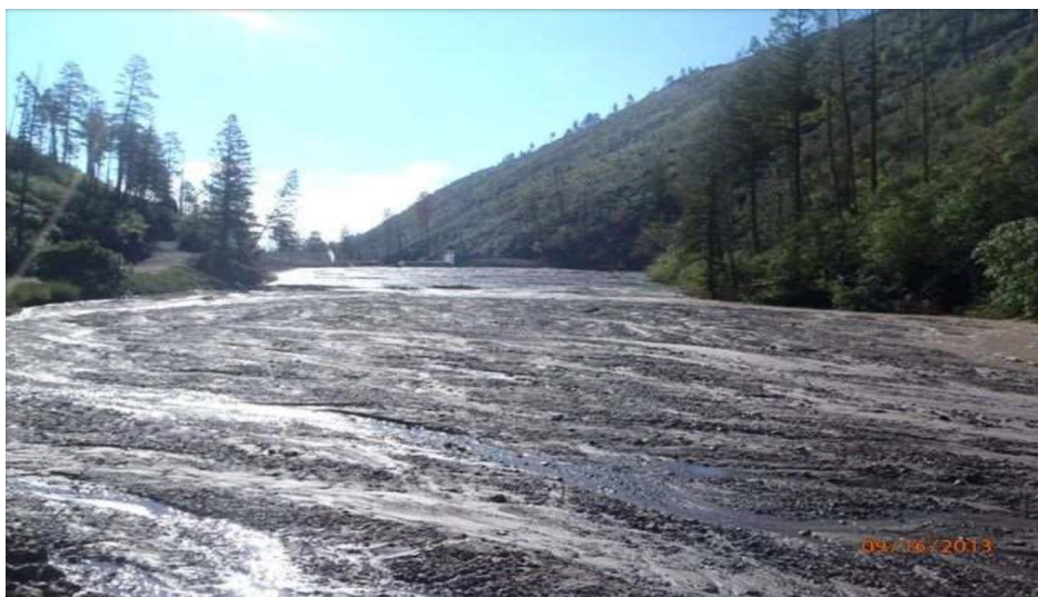
The aftermath of sedimentation into the newly restored Los Alamos reservoir following rain events over the burn area in summer 2013
